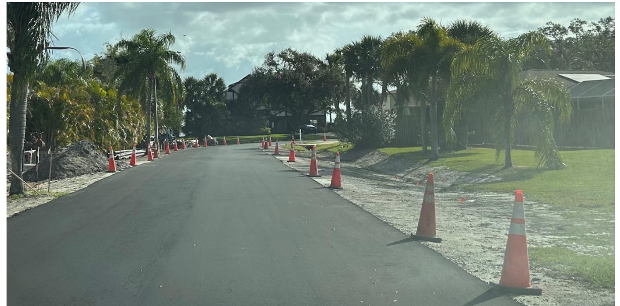
Construction of septic-to-sewer conversions in Suntree
