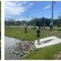
DAVID E. WEST PARK DETENTION POND OUTLET
