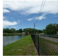
ELMER POND AT 80th AVE
