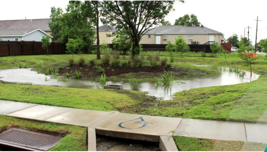
Reduced risk of flooding & damage
