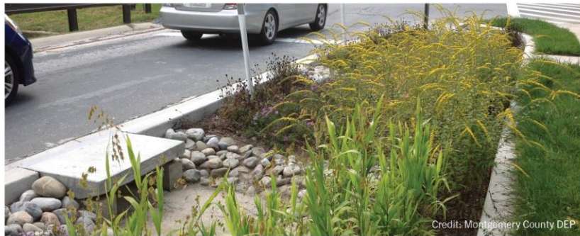
Credit: Montgomery County DEP
