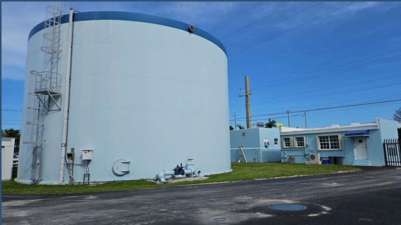
Pre-construction of FKAA – Marathon Pump Station Adaptation Project.
